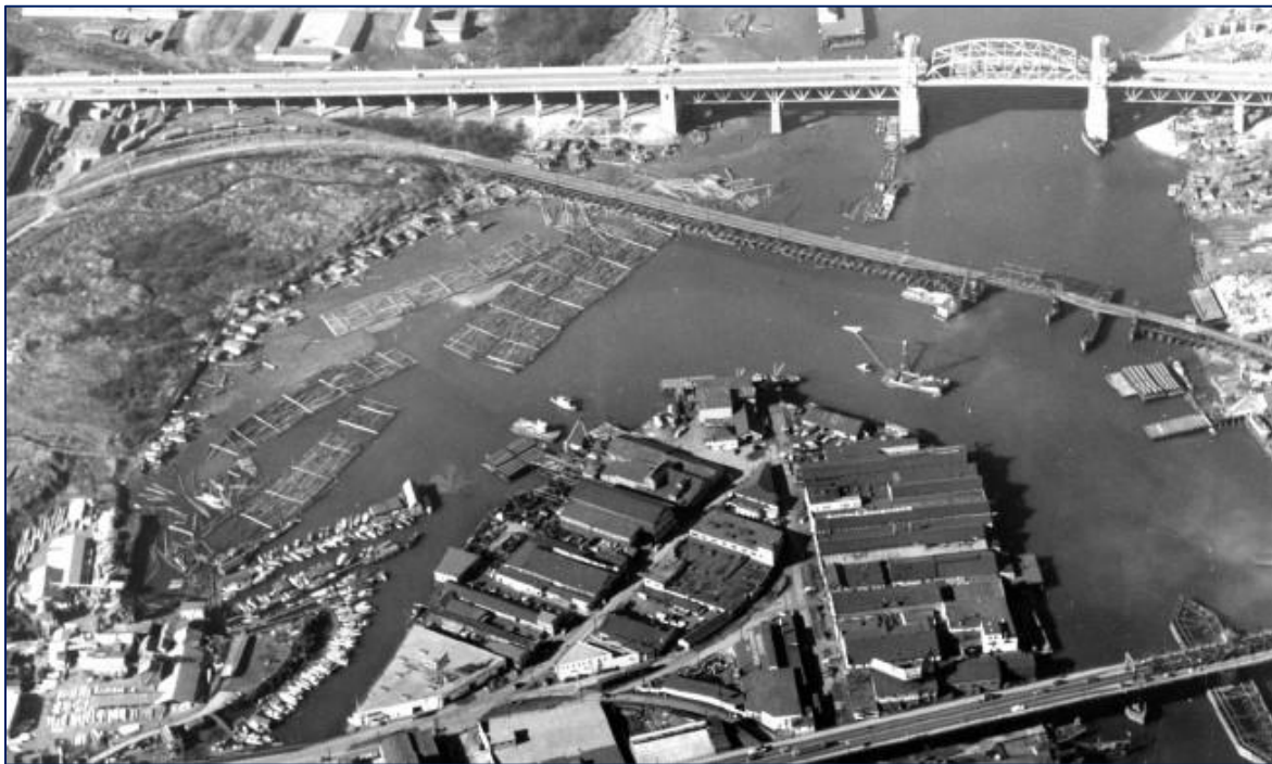
Burrard Bridge / Kits Trestle pivot-span bridge / Granville Bridge circa 1950
