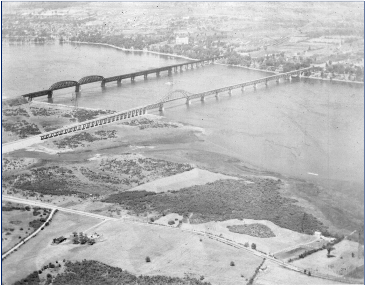
A view of the Honoré Mercier Bridge and Kahnawake, Que., prior to the construction of the St. Lawrence Seaway. (The Kahnawake Photo Archive/ Kanien'keháka Onkwawén:na Raotitióhkwa Language and Cultural Center)
